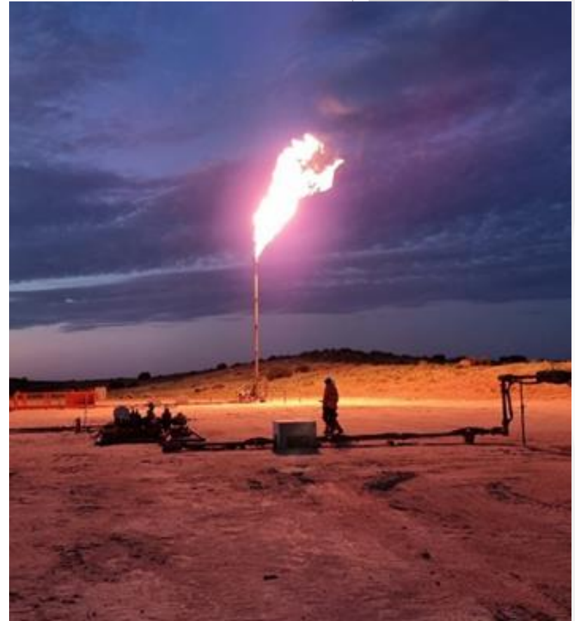
Figure 1: Gas flare from Kiwi-1 wellsite at 1.7 mmcf/d
