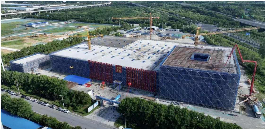
Photo: Vmoto's new manufacturing facilities in Nanjing, China under construction
